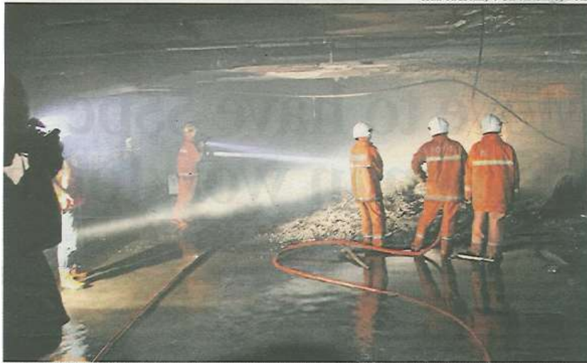
Firemen dousing fire on the ground floor of the New Central Mall in Jalan Tun Sambanthan yesterday.
